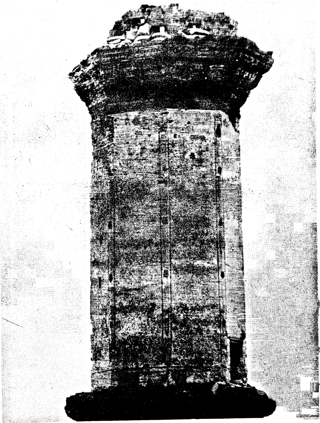
'Bunga' —A tower like minaret which was fortified completely and brought down heavy fire.
